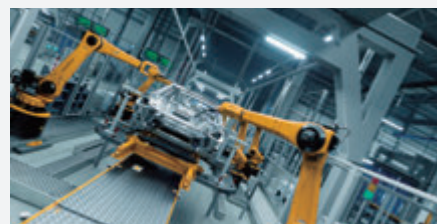
Supporting Accurate Inspection in Assembly Processes.
